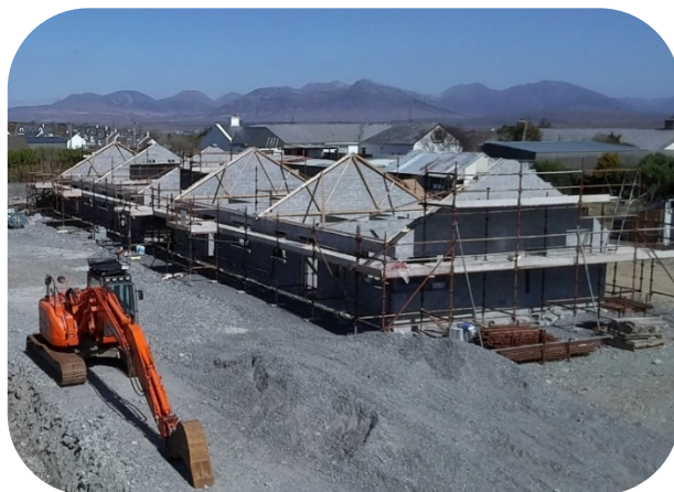
Delivering homes - construction underway: Cnoc na Carraige Roundstone
