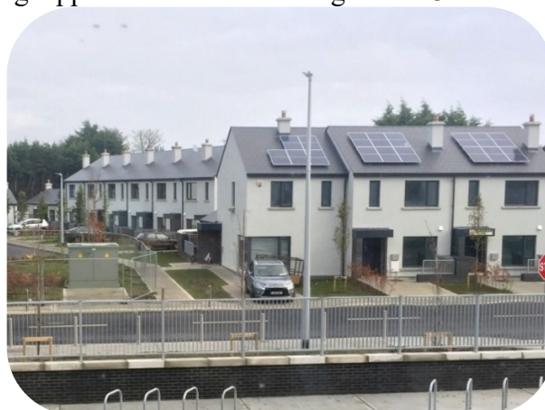
Delivering Homes – Building Communities: Cúil Ghréine, Tuam
