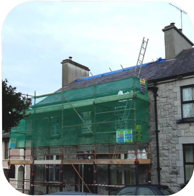
BHIS 19/17: Reslating of roof at Cross Street , Athenry
