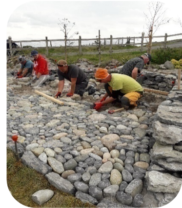
Stone Wall paving workshop
