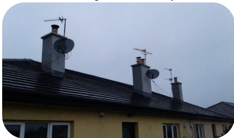
New Chimneys and Structural Roof Repairs at Creggane Traveller Specific Group Housing
