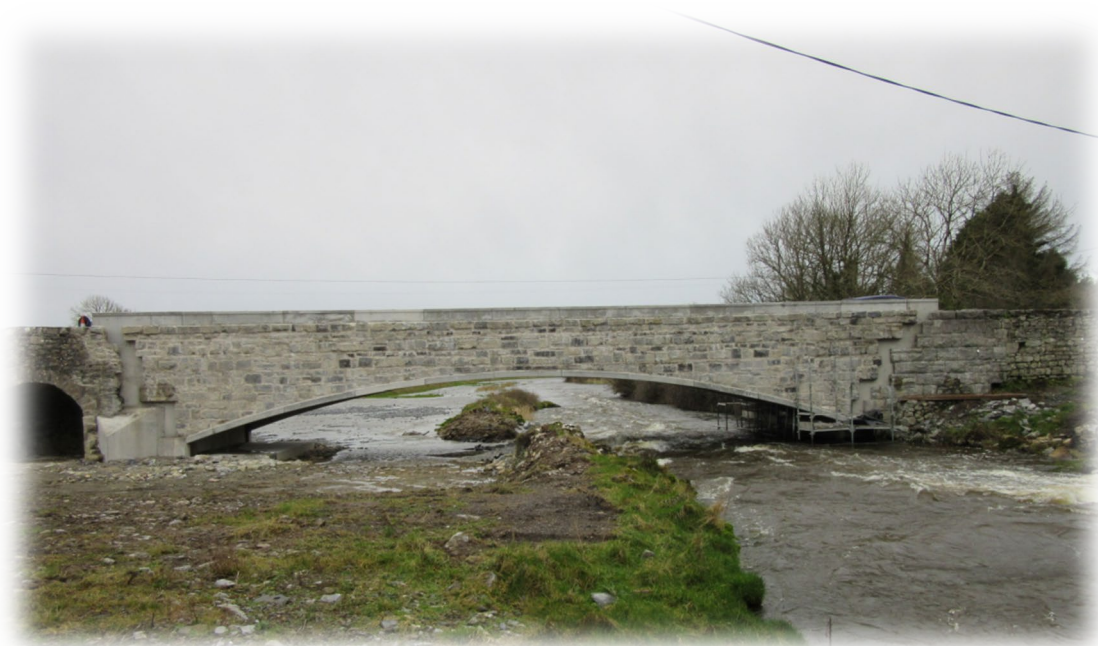
Dunkellin River & Aggard Stream Flood Relief Scheme – Newly constructed span at Dunkellin bridge
