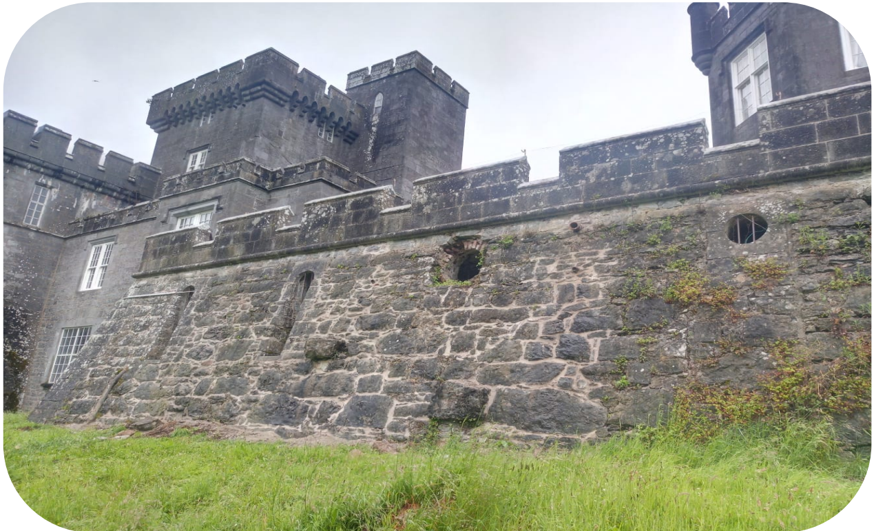
HSF 19/4: Lough Cutra stonework repairs with lime render mortar to stabilise terrace
