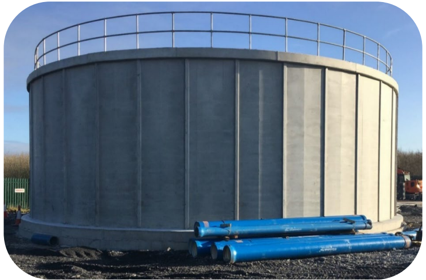
Completed 1,000m 3 capacity reservoir at Seefin.
