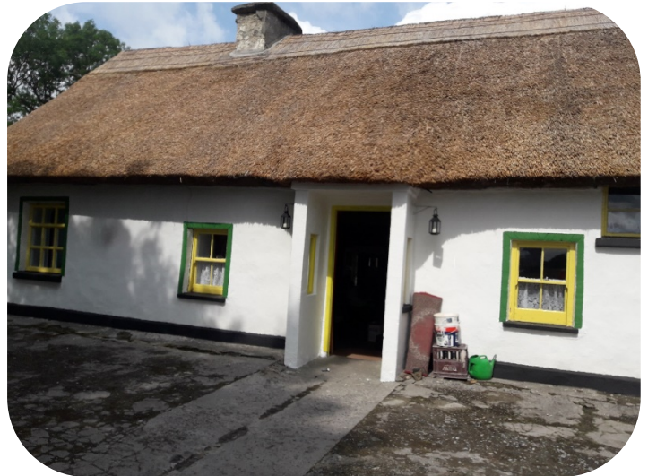
BHIS 19/20: Rethatch of roof of Keane's Cottage, Corrandulla
