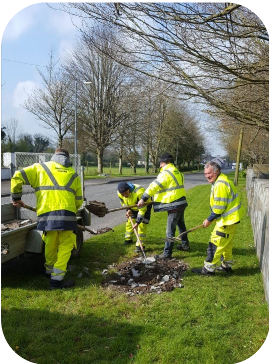
Works being carried out by Laurencetown/ Abbey Community Employment Scheme #YourCouncilDay
