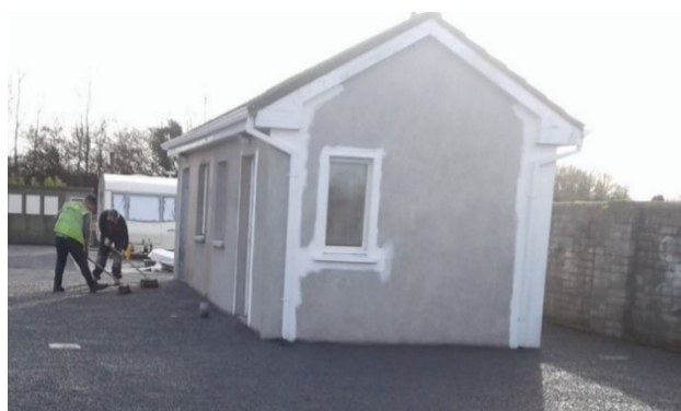
Additional Welfare unit and new surfacing at Capira Halting Site
