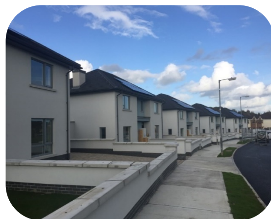
Building Sustainable Communities: Garbally Drive Ballinasloe
