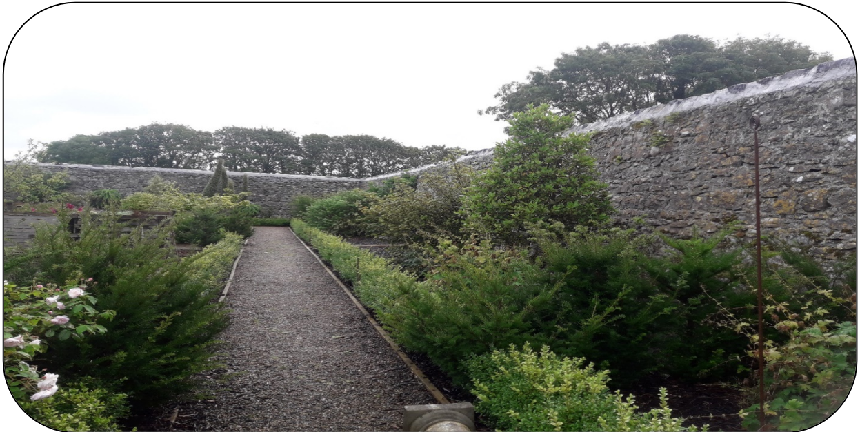
HSF 19/14: Duras Housewalled garden; repairs to capping of walls
