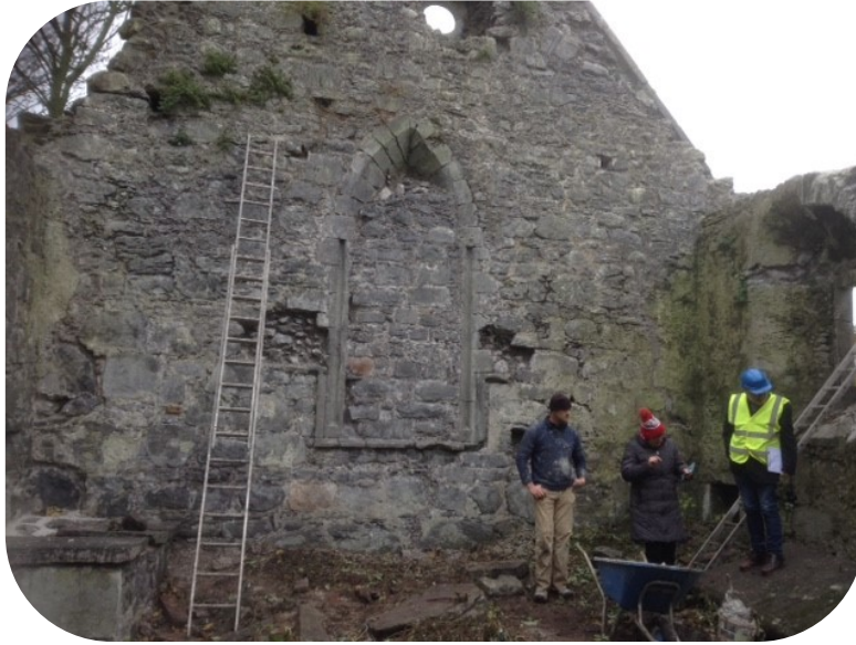
HSF 19/11: St Coman's Church, Kinvara, Co Galway – Final phase of works to consolidate the historic fabric completed.
